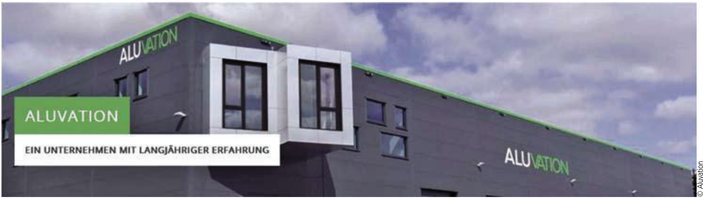
Abb. 1: Aluvation Technology Center ATC, Paderborn
